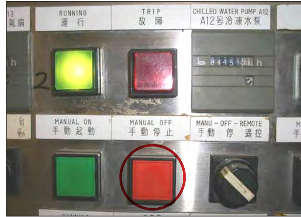
Photo 2 – For Chiller Water Pump #12 圖 2 – 凍水泵 #12
