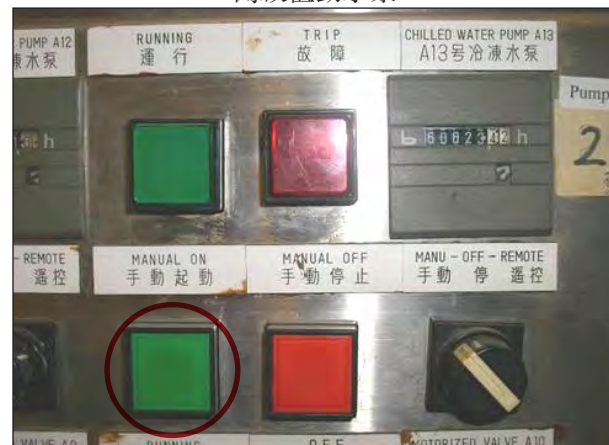
Photo 10 – For Chilled Water Valve #13 圖 10 – 凍水泵 #13
