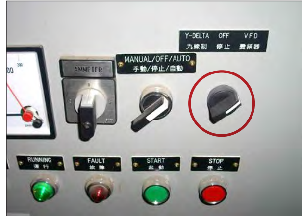
Photo 6 – For Water Pump #12 圖 6 – 凍水泵 #12
