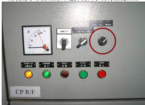
Photo 7 – For Water Pump #13 圖 7 – 凍水泵 #13
