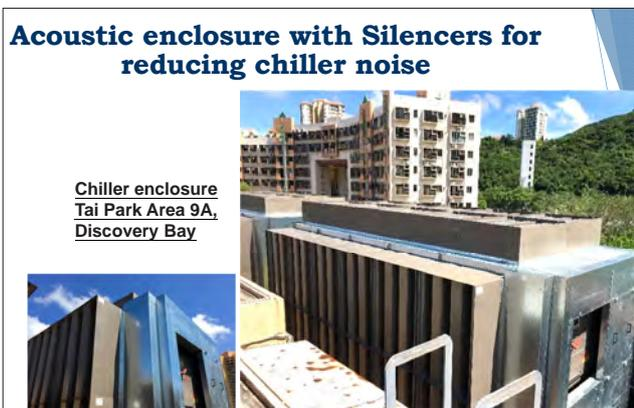
**Acoustic Enclosure for Air-cooled Chillers**
